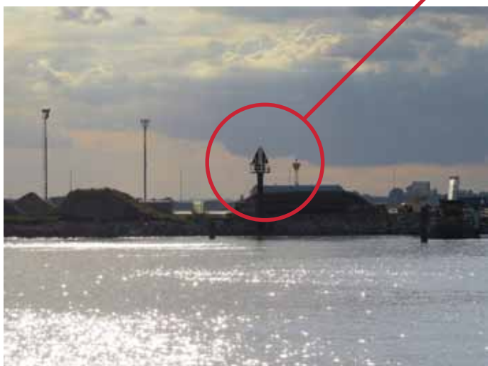
3 The shape and light of the transit triangles can be distinguished from the background of commercial port lighting and posts. At night, the forward light is sectored WRG.
