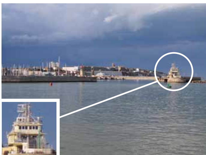
5 Traffic lights are displayed on top of the cream-painted port control building at the base of the northern breakwater ('3VG' to enter, or '3VR', no entry). If a flashing orange light is displayed, it means a ship is manoeuvring and you must not enter or leave harbour.
