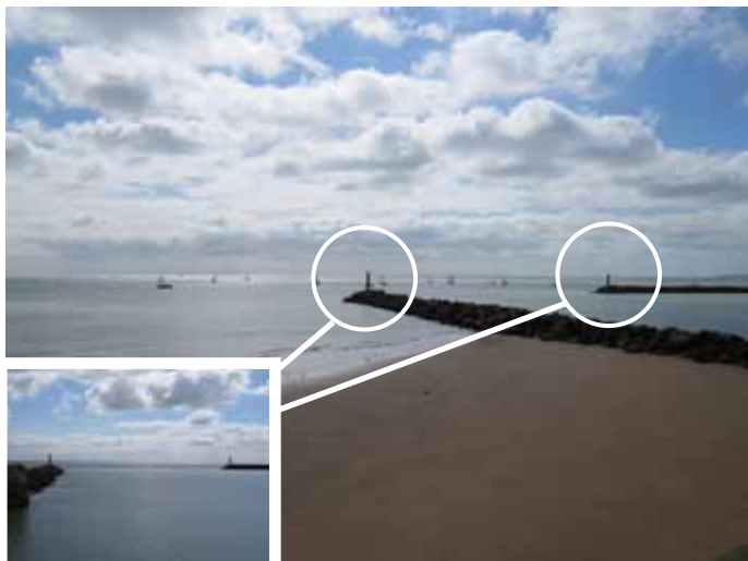
1 The outer breakwaters are marked with an Oc.G and a VQ.R on distinct beacons at the end of each wall.
